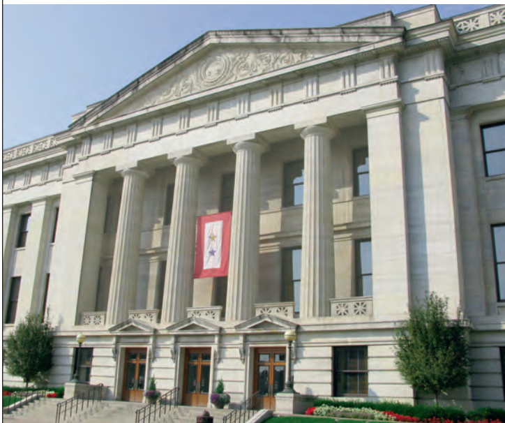
The rear facade of the Ohio Senate Building.
